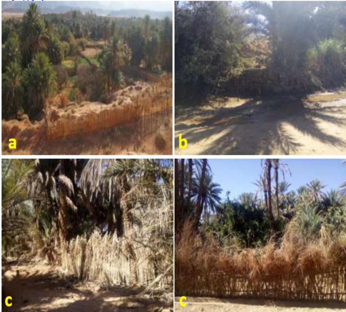
Figure 6. Windbreaks in the Boussemgoun oasis: a: ground wall; b: stone; c: dry palms
